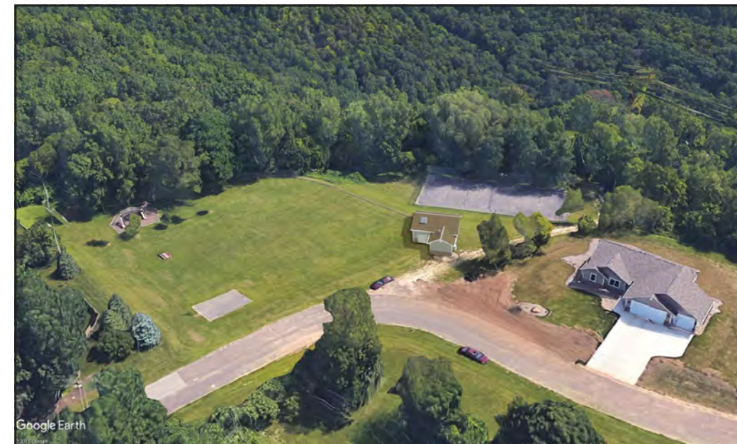
Briarwood Avenue Park with schematic of Well #2 well-house design and site layout.
